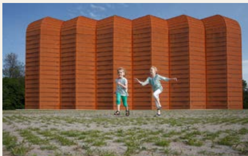
3.45 Science Park Amsterdam 150 kV station.
